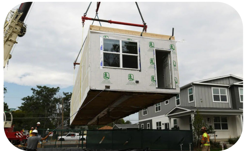
Image of a modular home construction
