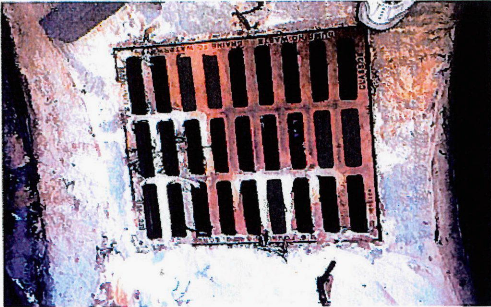
Photograph 1 – Facing south, catch basin with sediment washed in through silt fencing.
