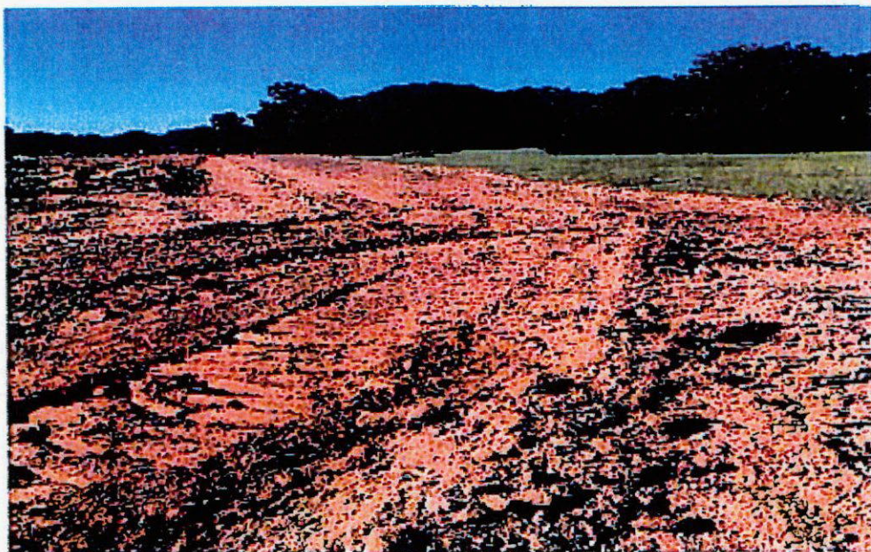
Photograph 4 – Facing southwest, west side of development without perimeter silt fencing.
