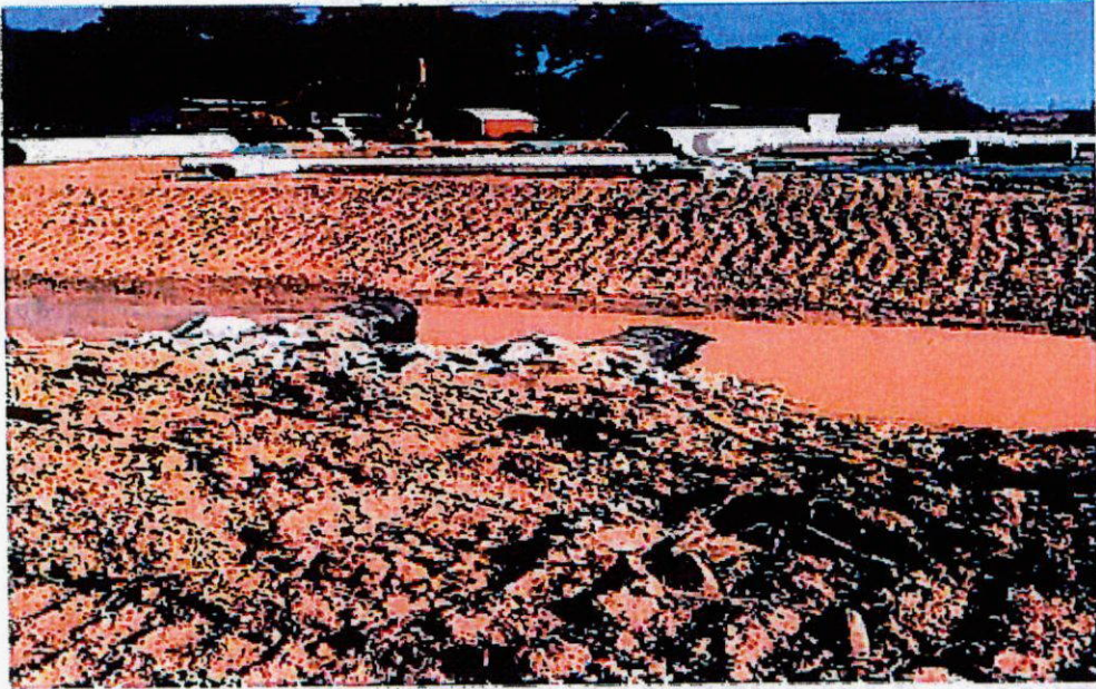
Photograph 9 – Facing north, Detention Pond banks require temporary/permanent stabilization.
