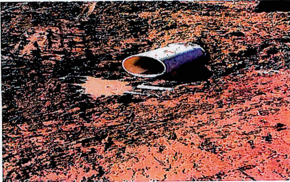
Photograph 11 – Facing south, culvert requires inlet protection.
