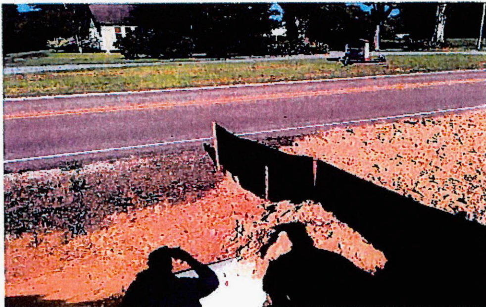
Photograph 8 – Facing northwest, entrance to development with inadequate controls between disturbed soils and highway drainage ditch.
